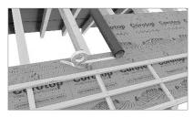
5. In order to eliminate draughts in the roof baffle, it is recommended (in case of roofs with pitches below 20° it is required) to bond the membrane overlaps with with the double-sided tape (e.g. Corotop Mix) or the adhesive strips integrated in the membrane and glued one to another (PLUS version).
