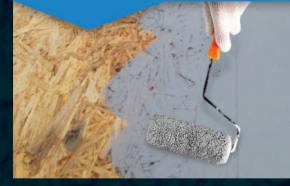
Apply a minimum 1-2mm Roof Seal coating and embed reinforcement matting into the wet coat.
