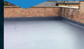
Finish with a further 1mm coat of Roof Seal to achieve minimum overall system thickness of 2mm.
