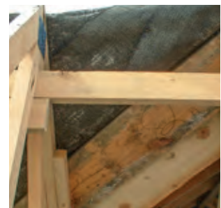
Mould damage because of trapped moisture
