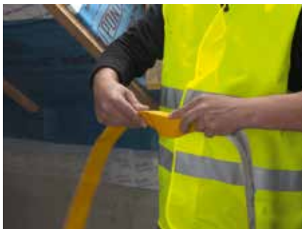
7. Fold Tyvek® Tape and remove smaller release liner strip
