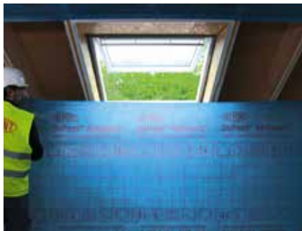
5. Measure required length of DuPont™ AirGuard® AVCL. Installation should start with the uppermost layer
