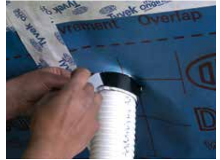
3. Remove the 2nd backing strip
