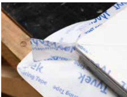
7. Form a loop on the corners: at least 1.5 x joint width - Repeat on all sides
