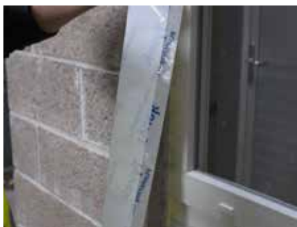
8. Fold a cut length of Tyvek® Plastering Tape and remove the narrow release strip
