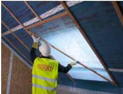
1. Cut a 'Y' into AVCL, using batten as a guide if preferred
