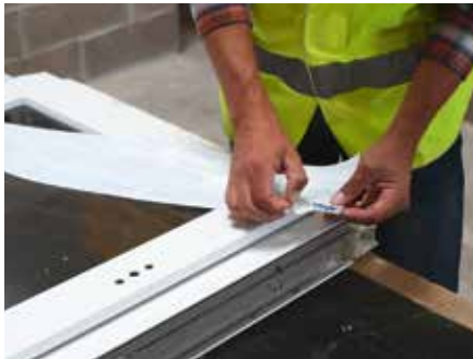
1. Using the 150mm Tyvek® Plastering Tape, start by removing the narrow release liner (20mm)
