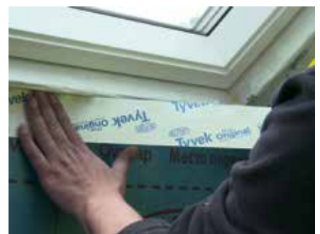
12. Seal tightly around window
