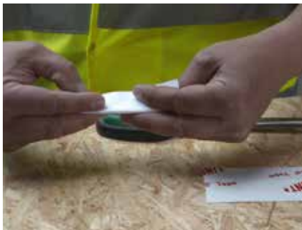
13. Fold DuPont™ AirGuard® Tape in half
