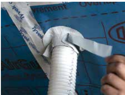
7. Once wrapped around, remove remaining release strip
