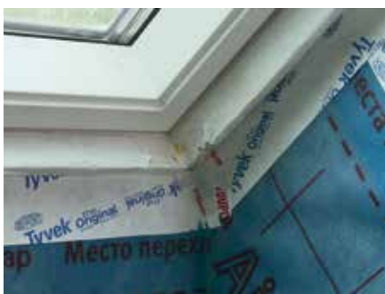
16. Cut tape may be used to seal internal corners
