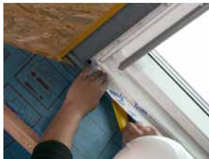
8. Bond tape to frame and remove remaining release paper
