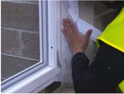
1. The internal window to wall junction can be sealed following the same method described on page 35
