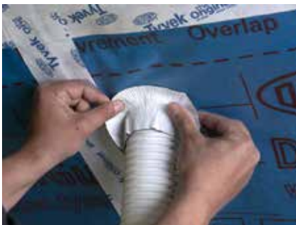
4. Fan the tape out onto the membrane, starting at the centre of the strip
