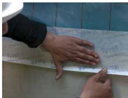
11. Cover equally the AVCL and the wall surface, removing each release liner in turn
