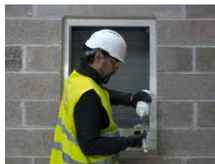
6. Tyvek® Primer can be applied onto the wall surface or directly onto the brush
