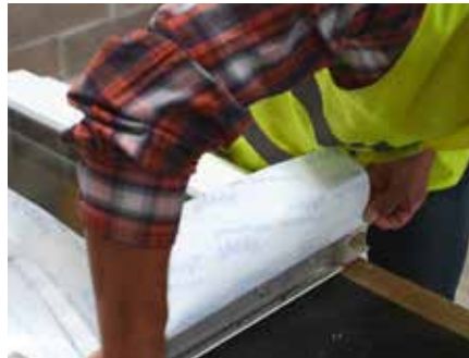
2. Fold the exposed tape strip back and apply to the frame
