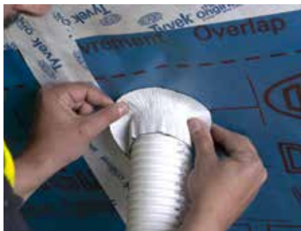
5. Press firmly to establish seal
