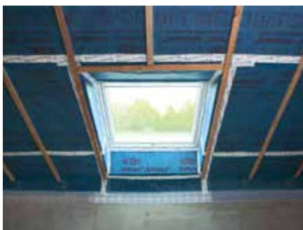
19. All sealing work can be easily checked by a visual inspection
