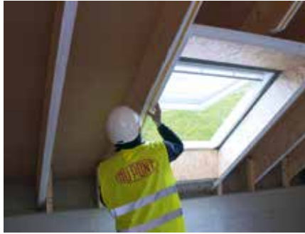
2. Apply tape to all facing surfaces . . .
