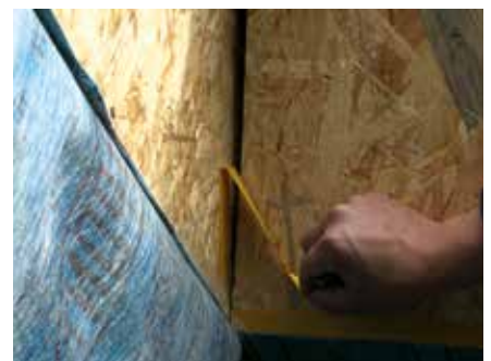
6. Remove release liner from DuPont™ Tyvek® Double-sided Tape (20mm) applied previously
