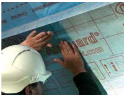
8. AVCL should be pressed firmly against tape
