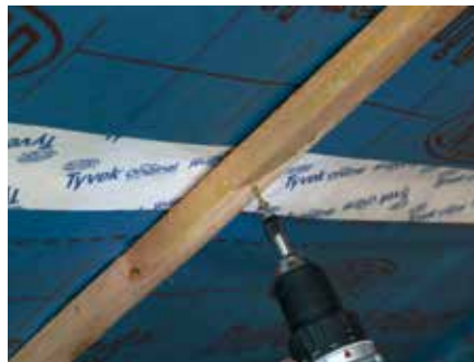
14. Press batten into position and permanently fix
