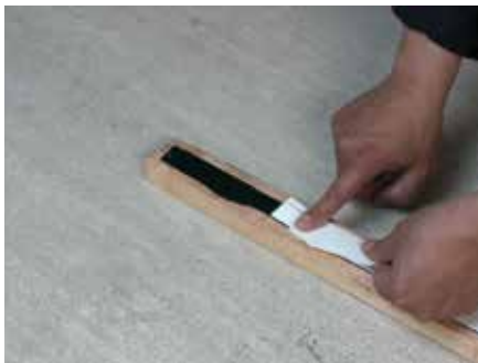
13. Remove release liner
