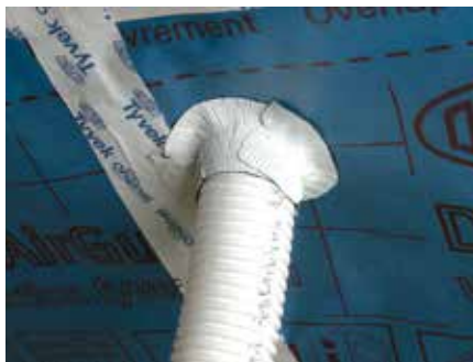
8. Make sure Tyvek® FlexWrap EZ is bonded to both the pipe & the AVCL
