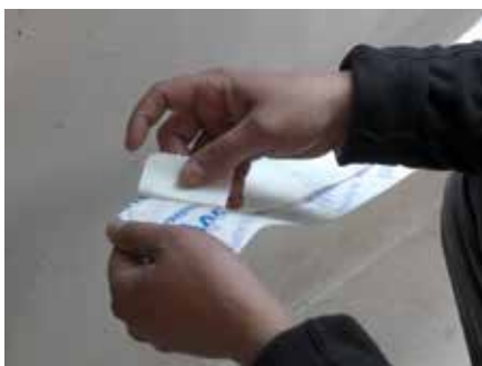
10. Peel away a short length of liner and apply the exposed tape onto the AVCL
