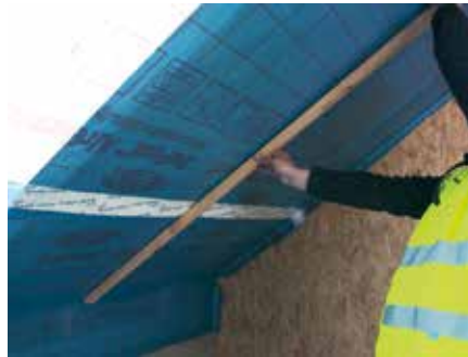
11. Measure battens prior to fixing
