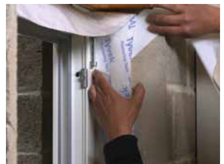
9. When the window unit is fixed into the opening remove the remaining release paper and apply Tyvek® Plastering tape on the interior side of the window. Finish as per page 36.
