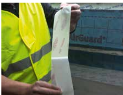
17. Remove release liner from DuPont™ AirGuard® Tape . . .
