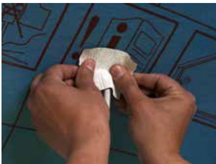
4. Remove one strip of release liner and bond to AVCL immediately adjacent to cable
