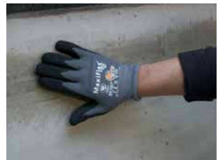
6. After an hour the primer turns transparent
