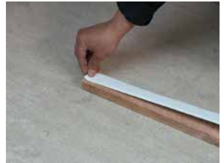
12. Apply Tyvek® Butyl tape to batten
