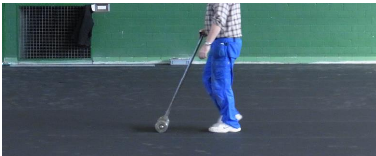
Figure 3: Pressure the installed SPORTEC® floor covering
