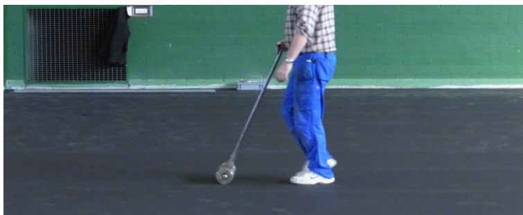
Figure 3: Pressure the installed SPORTEC® floor covering
