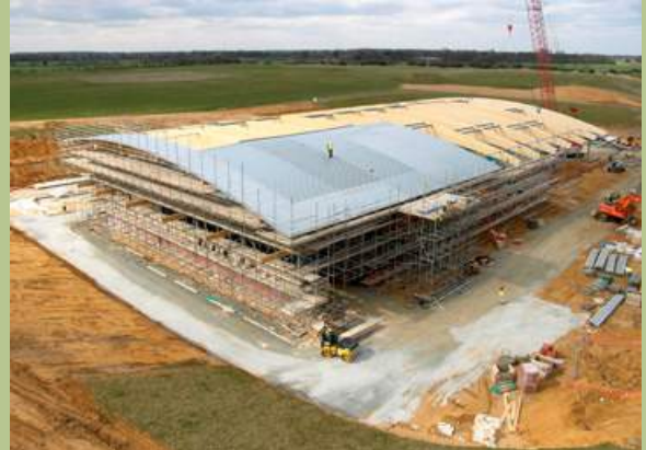
Roof covering installed
