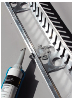
Tacking green roof retention
