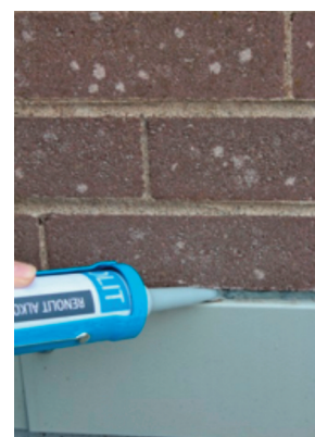
Sealing chased metal edge to RENOLIT ALKORPLAN onto a sacrificial layer
