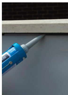
Sealing perimeter upstand
