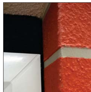
Fig 3 Head of frame after settlement - TP450 to head and TP601 to jamb
