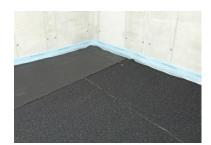
2. Place DAMTEC® system first and second layer over the entire surface to be covered. Trim to size slightly larger than the surface covered. Leave the underlay in place for 1 day (min. 24 hours) to allow dimensional relaxation and temperature equilibration.
