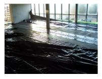
4. Cover underlay with PE membrane which should also cover the peripheral insulation strip and extend above the subsequent floor surface.
