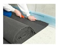
3. Use a Stanley knife to cut. Trim the underlay to the exact dimensions of the surface covered.
