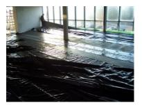
**1.** Before installation of floor system components, install a peripheral insulation strip over all structural components which extend upward or laterally such as walls, pipes etc.
