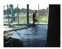
**5.** To avoid formation of sound conduction channels, be certain that screed cannot enter into the insulating underlay.
