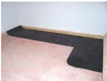
1. Sweep clean the existing dry concrete surface. Place the underlay **DAMTEC® 3D** over the entire surface to be covered. Trim to size slightly larger than the surface covered. Leave the underlay in place for one day to allow dimensional relaxation and temperature equilibration.
