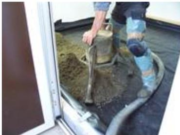
4. To avoid formation of sound conduction channels, be certain that screed cannot enter into the insulating underlay.
