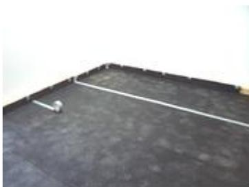
2. Use a regular carpet knife in conjunction with a steel straightedge for cutting **DAMTEC® 3D** to size. Install a peripheral insulation strip over all structural components (e.g. **DAMTEC® 3D**). Seal joints with high tack adhesive tape.
