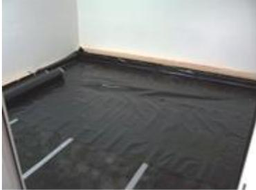
3. Cover underlay with PE membrane which should also cover the peripheral insulation strip and extend above the subsequent floor surface.
