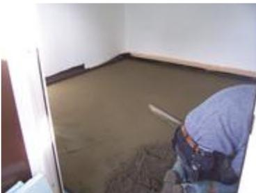
5. Install the screed or light weight cement. After finished installation start with floor finish. You can use other **DAMTEC®** products again for sound insulation.
