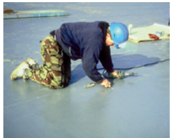
fig. 2: Verification of weld security
