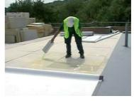
The membrane is then rolled back up again halfway or folded back and the adhesive is applied either by hand or by using an applicator trolley.
