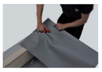
Cut away a section of membrane from the upstand strip.
