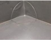
Hot air weld with a 20 mm nozzle in combination with a penny roller.
