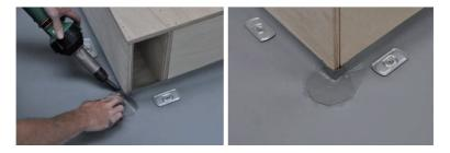
Cut an upstand strip of **RENOLIT** ALKORPLAN of the same height as the upstand to be waterproofed + 100 mm for the overlap with the field sheet.
