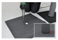
Weld the 20 mm lip using **RENOLIT** ALKORPLUS $_{81025}$  solvent and finish the seam with seam sealer.
