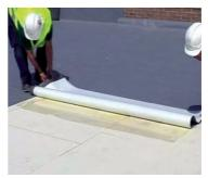
A **200 mm area free of glue** must be provided along end lap joints and at expansion or contraction gaps in the substrate.
