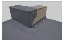
Weld the down the mitre fold to form a pocket. Weld inside the pocket working from the inside outwards
