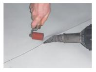
the nozzle of the gun, moving it back and forth, parallel to the nozzle and angled toward the seam.
