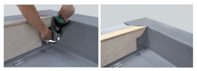
Follow the same procedure for the adjacent upstand. Cut the sheet into the corner as shown.
