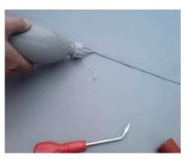
Ensure that the membrane is clean and dry before using seam sealer.
