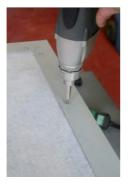
Cut the ALKORMETAL drip section so it fits onto an external corner and fix it to the substrate.
