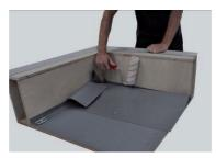
Weld up the fold to form a waterproof pocket. Work from the inside outwards.
