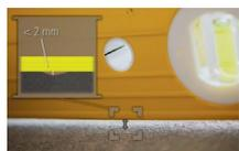
Unevenness of the subfloor may not be greater than 2mm measured over a width of 200cm.
