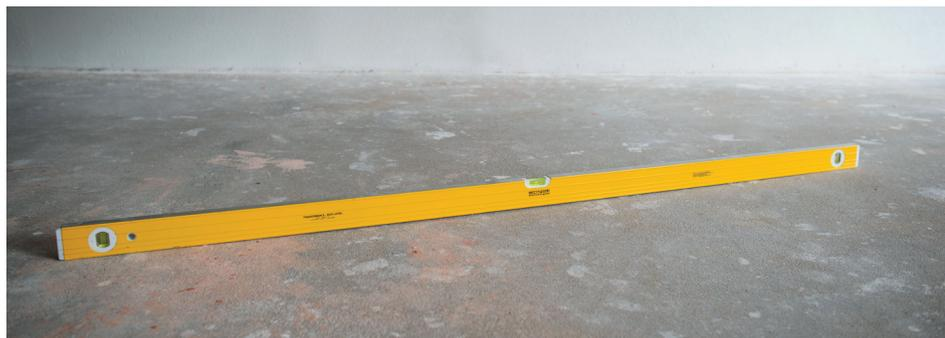
The subfloor must be hard, smooth, clean and dry, as well as being free from defects and fit for purpose. When required, scrape off and remove old adhesives and loose laying levelling compound. Make sure the subfloor is flat and free from chemical substances and other contamination.
