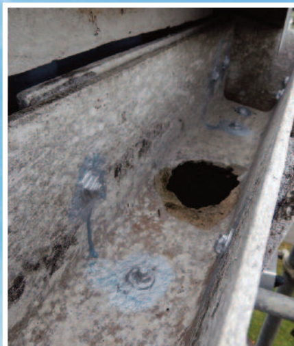
2 Corrosion treatment to fixings
