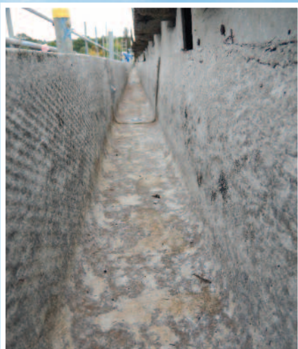
1 Cleaned, dry gutter
