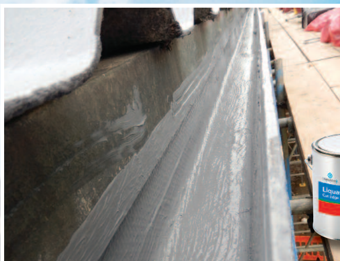
4 Finished seamless gutter lining
