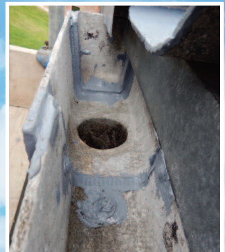
3 Gaps, joints and fixings coated with Non-Sag Sealer
