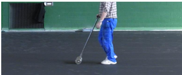
Figure 3: Pressure the installed SPORTEC® floor covering
