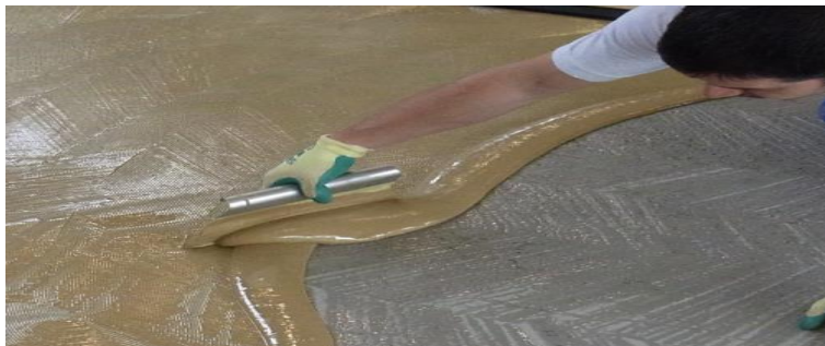
Figure 1: Glue application on the clean and leveled substrate
