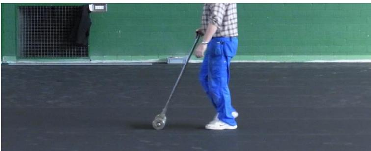
**Figure 3:** Pressure the installed **SPORTEC®** floor covering
