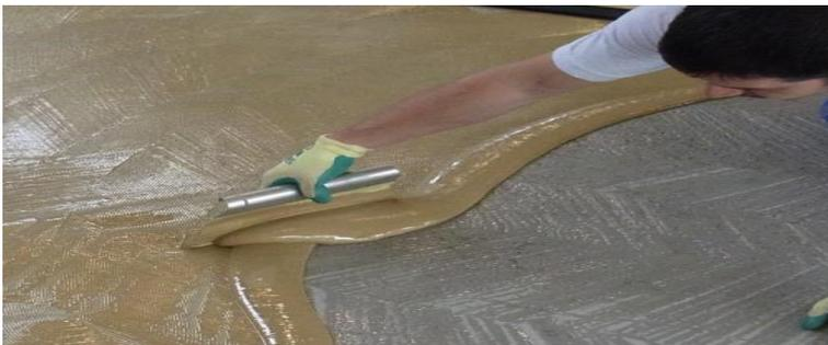
**Figure 1:** Glue application on the clean and leveled substrate
