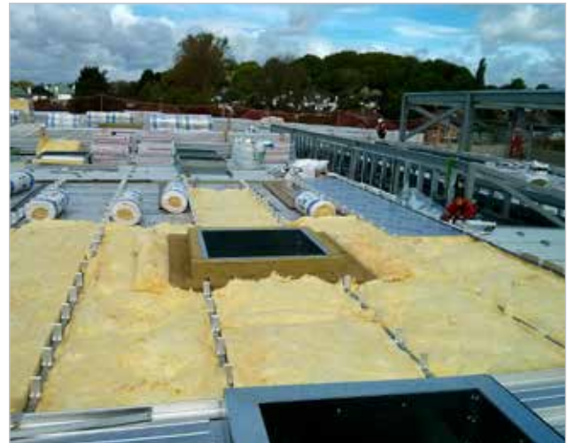
Soaker with rigid insulation in place
