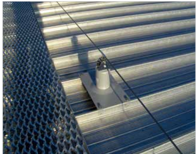
Walkway connection via Seam Clamp
