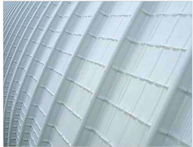
Dublin Port Tunnel
