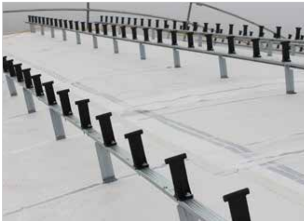
Triumph Activation, Barnwood Construction
