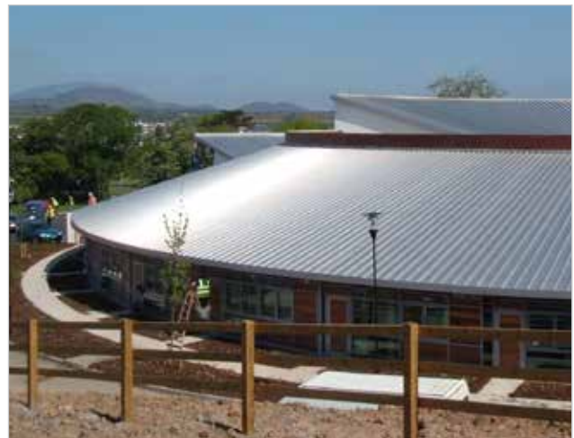
Sisters of Mercy, McNamara Construction
