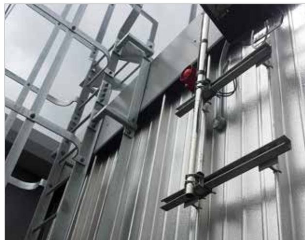
Accessories connected via seam clamps
