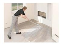
The substrate must be levelled and clean. If necessary use levelling compounds or primers. Check the usage instructions of the adhesive manufacturer for possible special procedures to follow over levelling compounds or primers if used.
