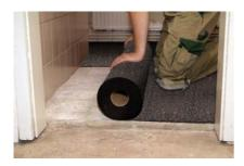
3. Place **DAMTEC®** standard over the entire surface to be covered. Trim to size slightly larger than the surface covered. Leave the underlay in place for one day to allow dimensional relaxation and temperature equilibration.
