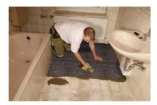
6. Put in DAMTEC® standard without fold and rub and press carefully. For the second half work in same way.
