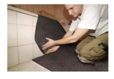
4. Trim **DAMTEC®** standard to the exact dimensions of the surface covered.
