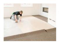
4. Fold back **DAMTEC®** standard to the middle of the room and glue the underlay to the substrate, observing the instructions of the adhesive and floor finish manufacturers.
