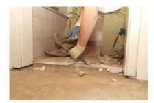
1. Remove old and loose tiles if necessary. The substrate must be levelled and clean.
