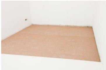
2. Place **DAMTEC® resistant cork (G)** over the entire surface to be covered, laying it perpendicular to the subsequent laying direction of the floor finish. Leave the underlay in place for one day to allow dimensional relaxation and temperature equilibration.
