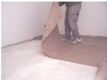
3. Fold back **DAMTEC® resistant cork (G)** to the middle of the room and glue the underlay to the substrate, observing the instructions of the adhesive and floor finish manufacturers. It's recommended to vacuum the floor once again before applying the adhesive. The ground side must be above after installation.
