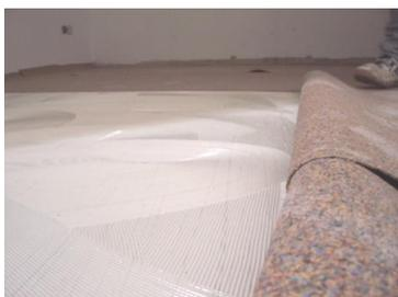
4. Put in **DAMTEC® resistant cork G** with the not ground side or **DAMTEC® resistant cork** without fold and rub and roll carefully.
