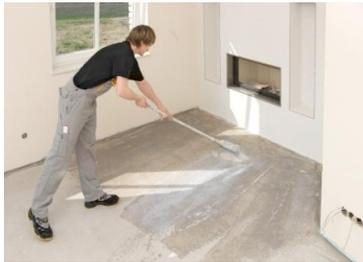
1. The substrate must be levelled and clean. If necessary use levelling compounds or primers. Check the usage instructions of the adhesive manufacturer for possible special procedures to follow over levelling compounds or primers if used.
