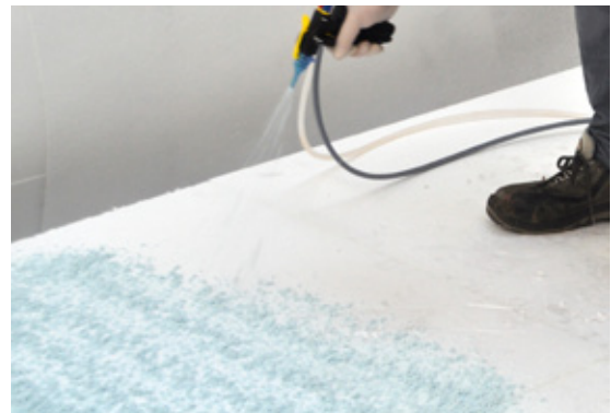
Pict. 2: The adhesive RENOLIT ALKORPLUS 81065 is atomized by means of a spray gun.
