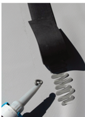
Isolating EPDM weather strips onto a sacrificial layer*
