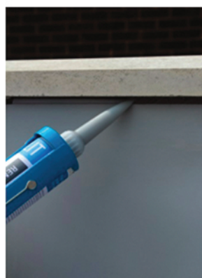
Sealing perimeter upstand
