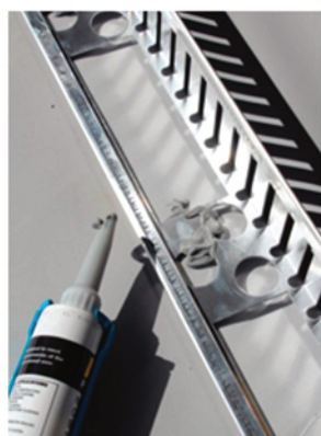
Tacking green roof retention
