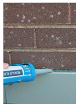
Sealing chased metal edge to RENOLIT ALKORPLAN
